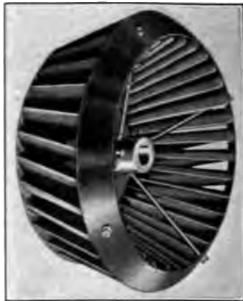
FIG. 121.—Runner of conoidal fan, Buffalo Forge Co.
